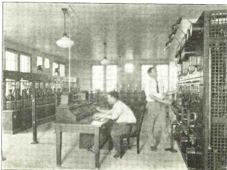
J. J. BELOUNGY (SEATED), ENGINEER-IN-CHARGE OF THE N. B. C. TRANSMITTER AT BELLMORE, L. I., AT THE RADIO RECEIVING SET TUNED AT ALL TIMES TO 600 METERS FOR "SOS" WATCH
